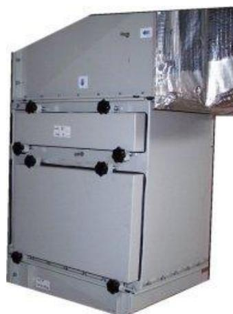
***Figure 6: Safe change filter housing mounted externally***
